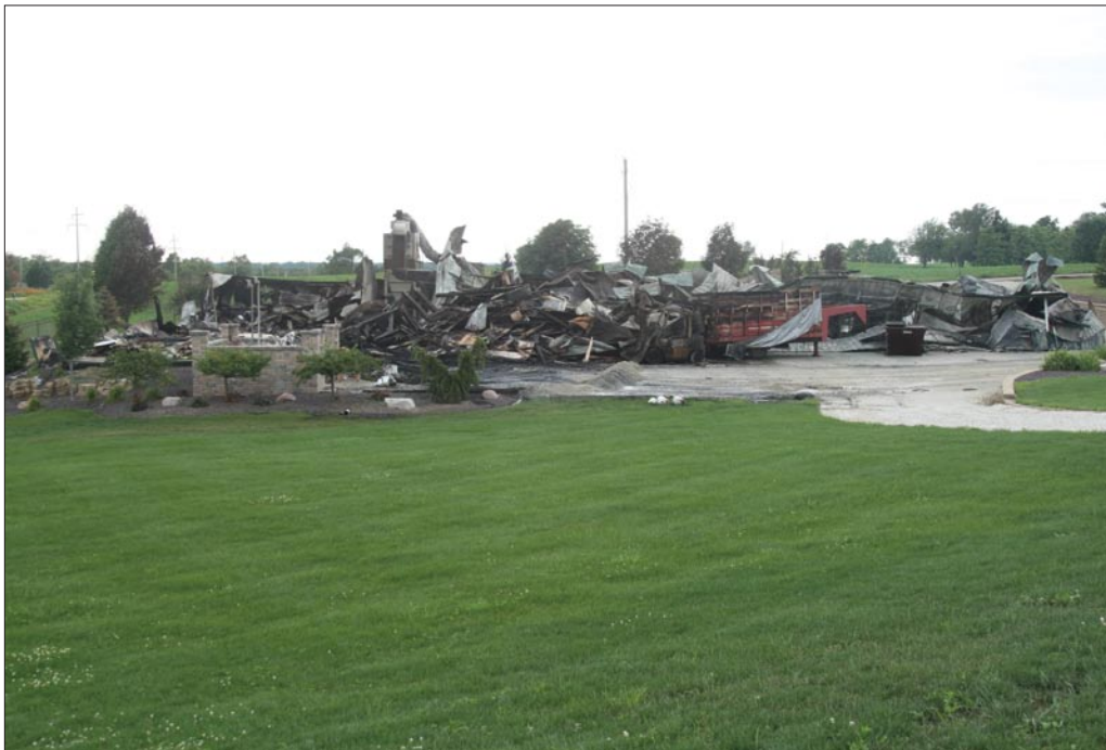
The company lost nearly everything in the fire (above), with not one piece of machinery able to be salvaged.
